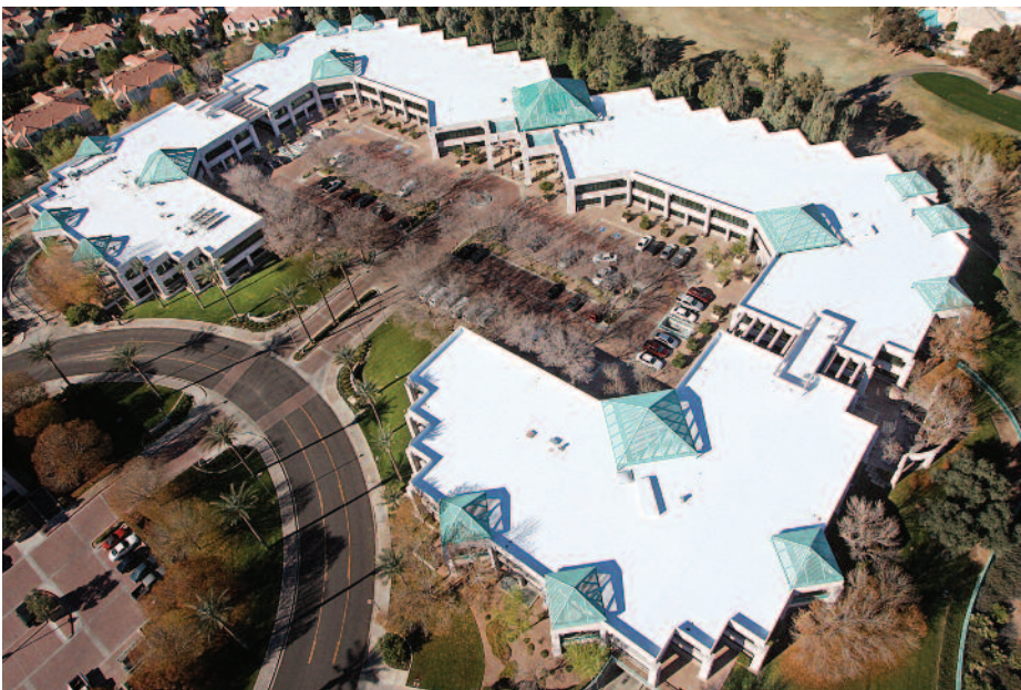
The Nationwide Scottsdale Insurance building before (top) and after (bottom) Starkweather Roofing installed the cool roof system
